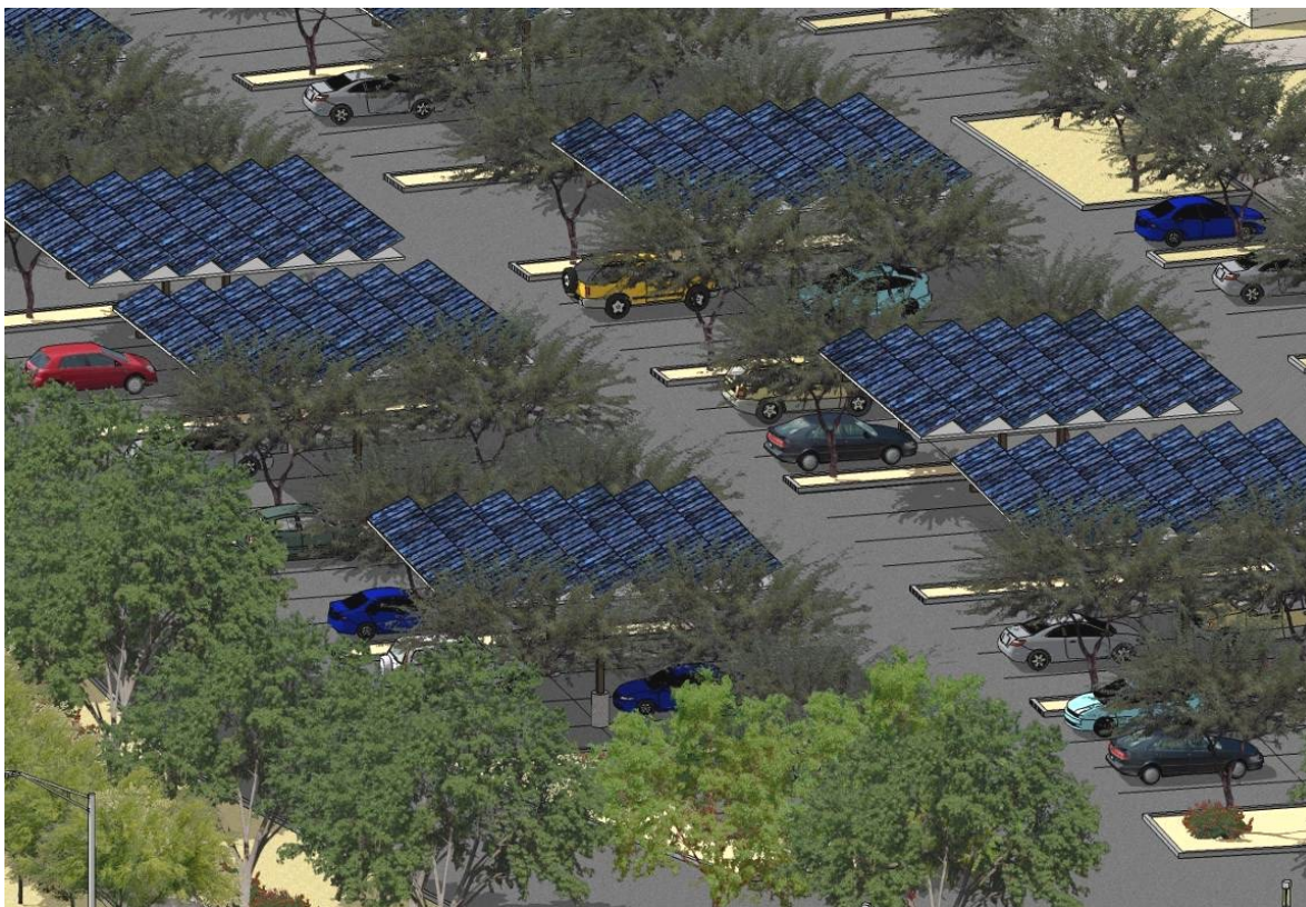
Figure 22: Parking Shade Structures Including Solar Panels
