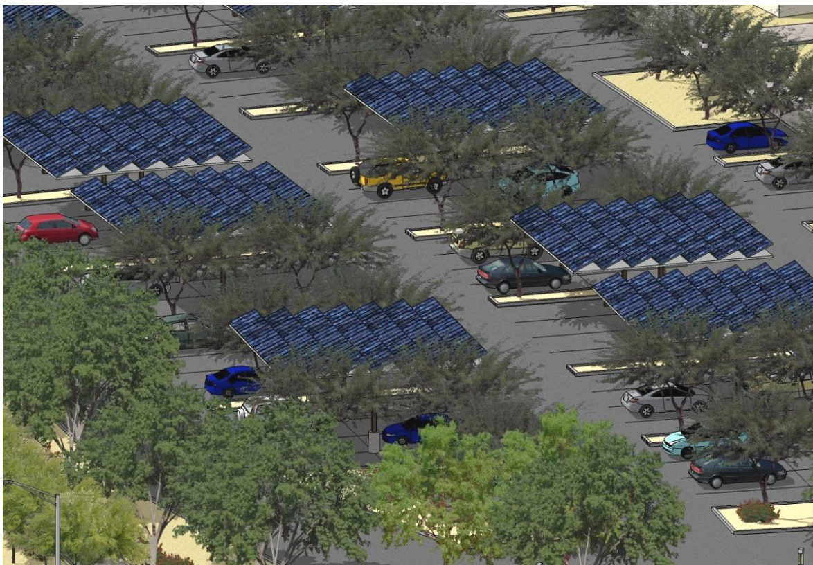
Figure 23: Parking Shade Structures Including Solar Panels
