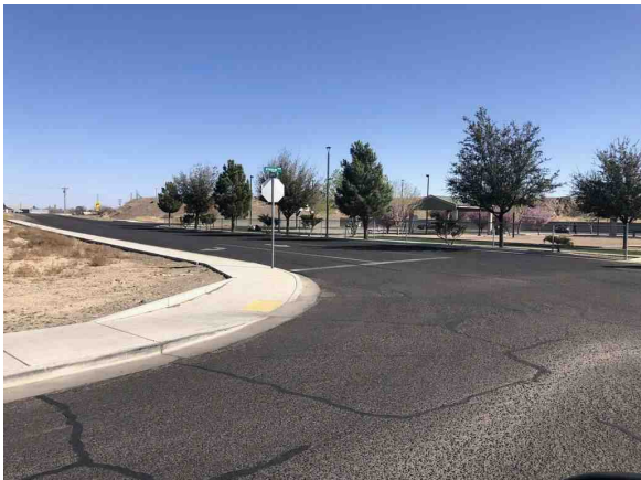
Street South Side
